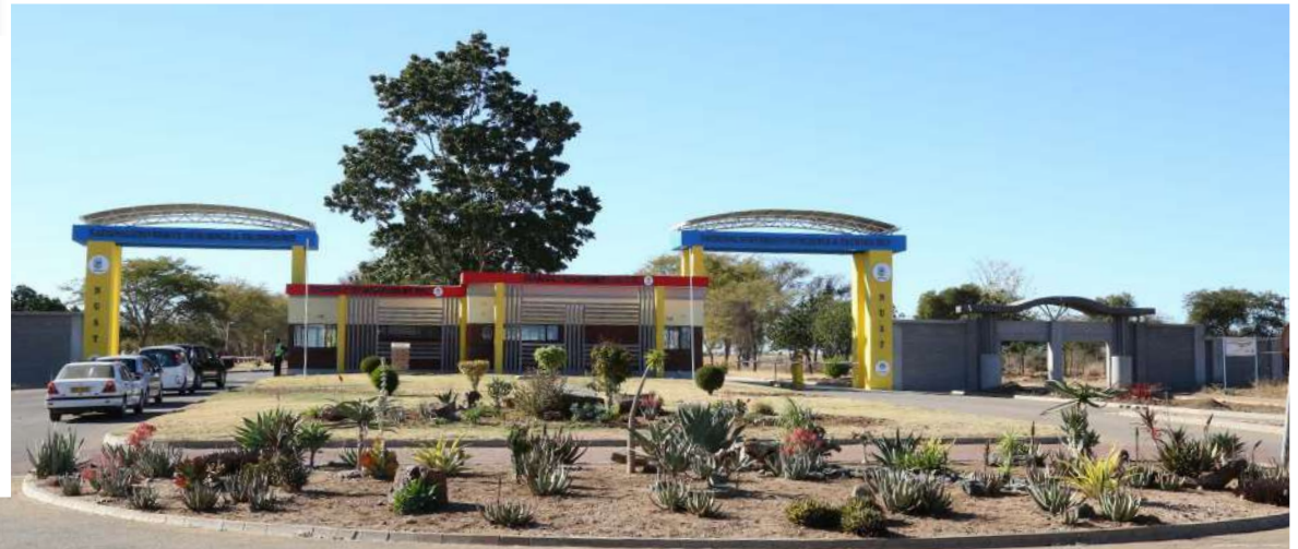
The new Nust Gate house which was constructed with the help of PPC.
